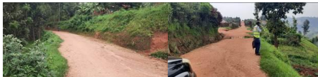
Figure 3: Typical roads of the project areas.
